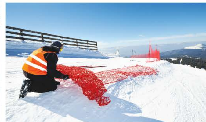
Protective net installation
